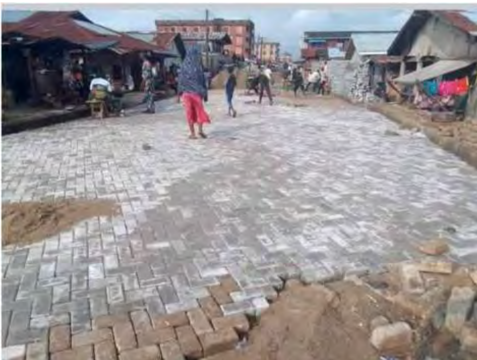
Akorede Road in progress
